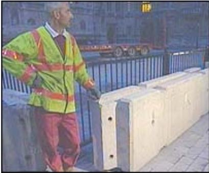
Concrete blocks. Cheap, simple and robust, such blocks were put out around Westminster Square as a first line of defence when the current increased threat level first emerged. They do help as a physical barrier against forced entry by vehicle but given a large enough device, would act as rather large secondary projectiles. Would work better if anchored to the ground and to each other. They are also good in a multi-hit environment for both blast and ballistic threats.
