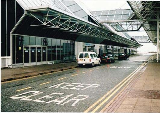
Large glass frontage with cars able to park within a few feet. Even with the rigorous Police presence employed at an airport it would be easy for a Vehicle Borne IED to be used, especially as a suicide bomb. The lower elevation was similarly glazed with added benefit to the bomber of greater confinement, reflection surfaces and all the things you don't want to have to protect against.
